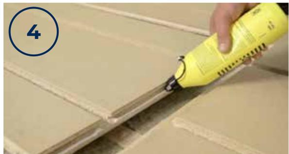
The boards should always be glued to each other at the tongue and the groove. The boards can also be glued to the base to avoid possible creaking. The glue should be an appropriate PVA wood glue. Application of the glue should be done carefully ensuring that there is a continuous seam of adhesive along the entire length of the tongue and groove. Note however that excessive use of glue might lead to gaps between the boards.
