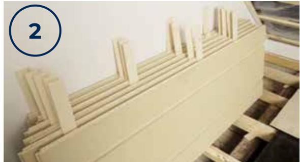
Before installation, the moisture content of the KoskiTherm boards should be stabilized close to the conditions of use. The boards should be stabilized for 5-7 days, depending on the initial moisture content. The boards should be separated with battens whilst being stabilized.
