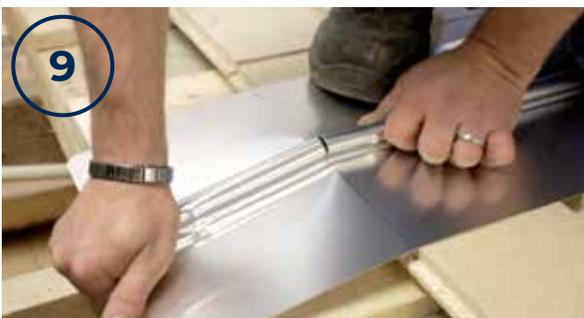
Use the folding points to cut the plates to the correct measure. Straighten any bent corners of the plates before installation.
